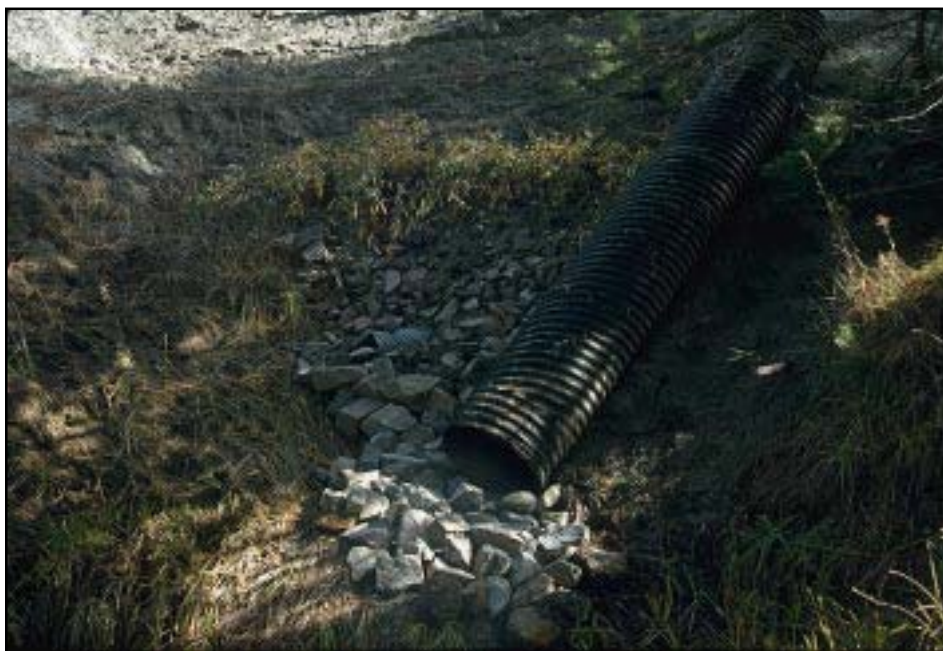
Photo 8.1 Protect the outlet of culverts against erosion. Graded riprap is common used for this purpose.
