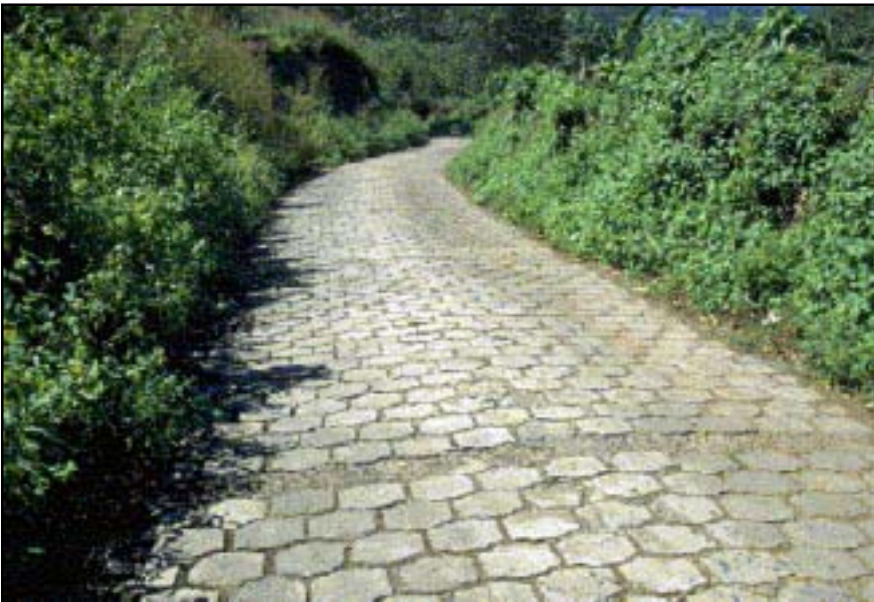
Photo 12.7 Concrete blocks (Adoquin) or cobblestone offer an intermediate alternative to aggregate and pavement road surfacing. These materials are labor intensive to construct and maintain, but are very cost-effective in many areas.
