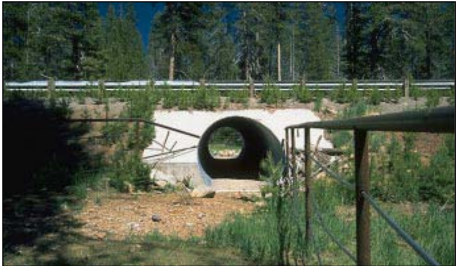
Photo 2.7 A road underpass constructed to allow animals to move safely from one side of the highway to the other.
