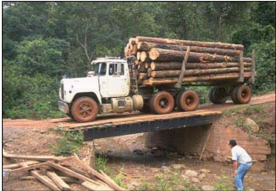
Photo 10.1 Culverts, fords, or bridges may be used for stream crossings. Use bridges to cross large permanent streams, minimize channel disturbance, and to minimize traffic delays. Use an opening wide enough to avoid constricting the natural channel. Locate the bridge foundation on bedrock or at an elevation below the anticipated depth of scour.
