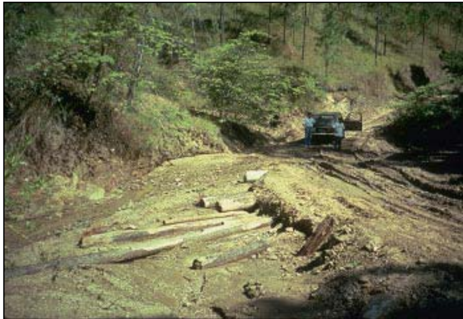
Photo 8.10 Most log culverts have very little flow capacity. Remove temporary log (Humboldt) culverts before major rainstorms or before the rainy season.
