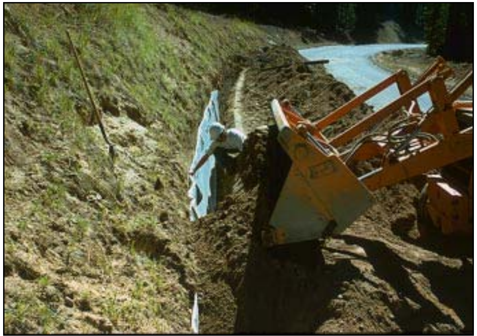
Photo 6.4 Use of geotextiles placed against fine soil to provide adequate filtration for an underdrain.
