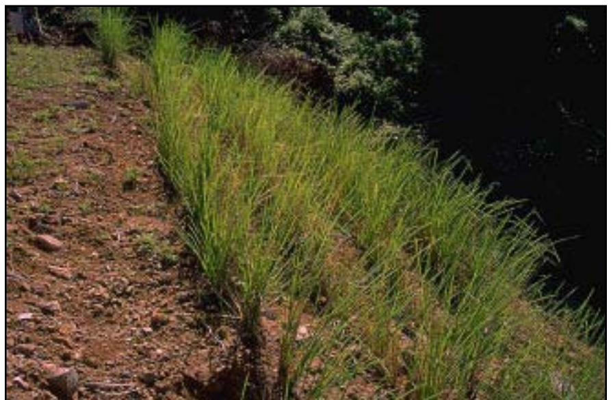
Photo 13.9 Use of Vetiver grass for slope stabilization and erosion control. Choose vegetation that is adapted to the site, has strong roots, and provides good ground cover. Ideally, use native species.
