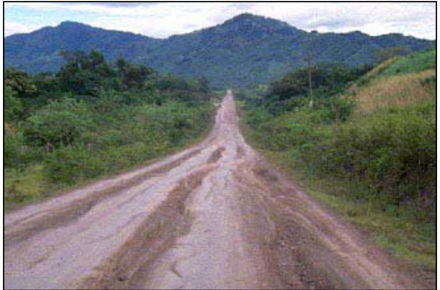
Photo 12.3 A road in need of maintenance and surfacing. Add roadway surface stabilization or do maintenance with grading and shaping of the surface to remove ruts and potholes before significant road damage occurs, to achieve good road surface drainage, and to define the roadbed.
