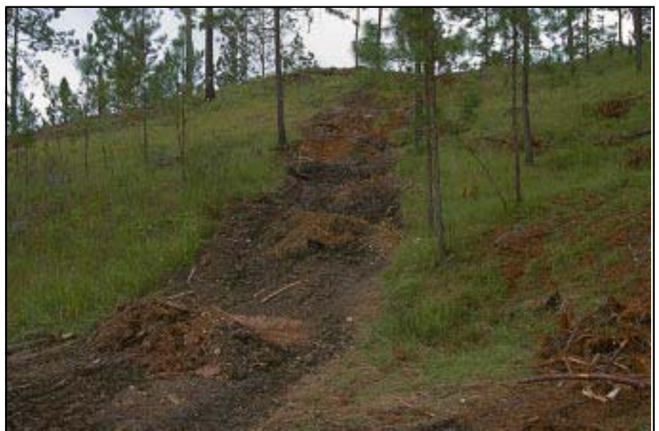
Photo 3.8 Stabilize skid roads and trails after use with water bars and apply a ground cover or other erosion control measures.
