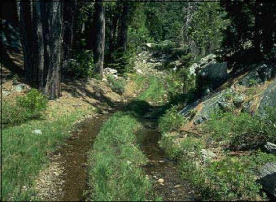
Photo 3.2 A poor road location where the road has become a “creek” and is hydrologically “connected” to streams around it.
