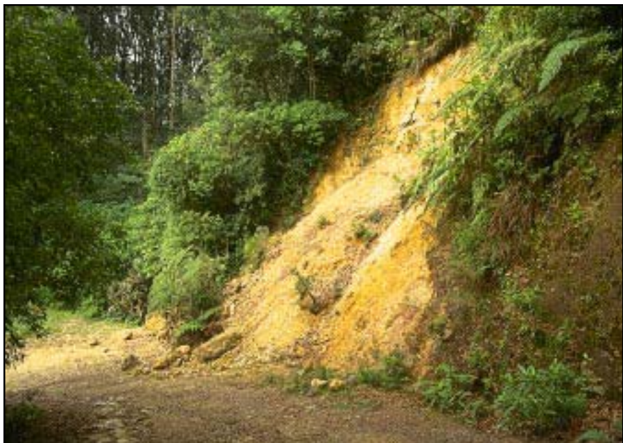
Photo 11.1 Over-steep slopes, wet areas, or existing slide areas can cause instability problems for a road and increase repair and maintenance costs, as well as sediment production.
