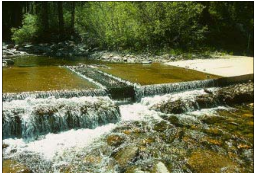
Photo 9.4 Use vented fords with pipes or openings to keep traffic out of the water most of the time, minimize traffic delays, and allow for fish passage. Note the downstream scour protection with gabions and rock.
