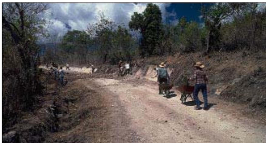
Photo 4.7 Use the road construction techniques that are most appropriate and cost-effective for the job and geographic area. Hand labor versus equipment depends on labor costs, equipment availability, and production rates.
