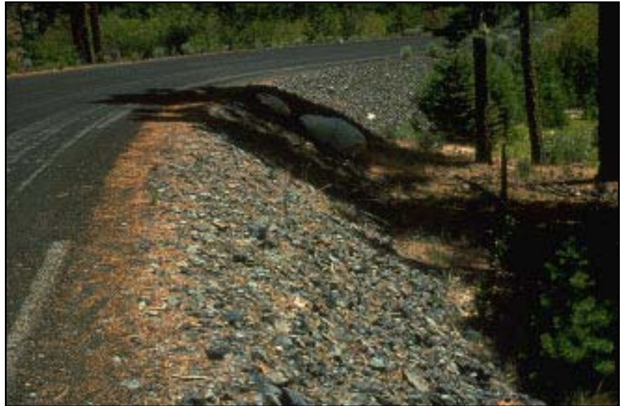
Photo 13.7 Rock armoring, placed on a very erosive soil fill slope adjacent to a creek, used for durable, permanent erosion control.
