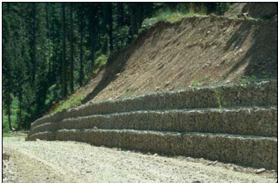
Photo 11.9 Gabions are a commonly used type of low gravity retaining structure because they use locally available rock and are relatively inexpensive.
