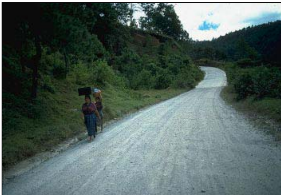
Photo 1.1 A minimum impact rural road that is well drained, has a stable driving surface, stable slopes, and is satisfactory for the user.
