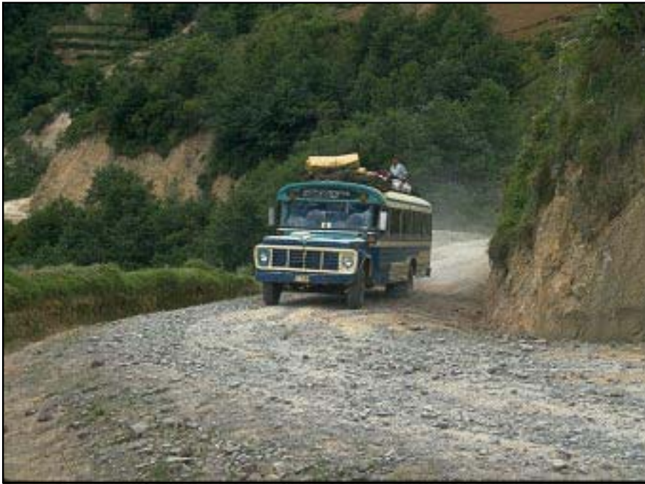
Photo 3.1 A low-volume, local road, with minimum adverse environmental impact, that serves local users by providing access between communities.
