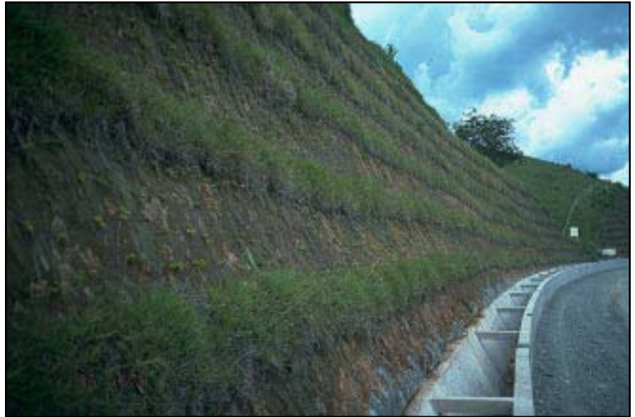
Photo 13.10 Use of grasses, planted on contour, to provide surface slope stabilization and erosion control on a steep road cut.
